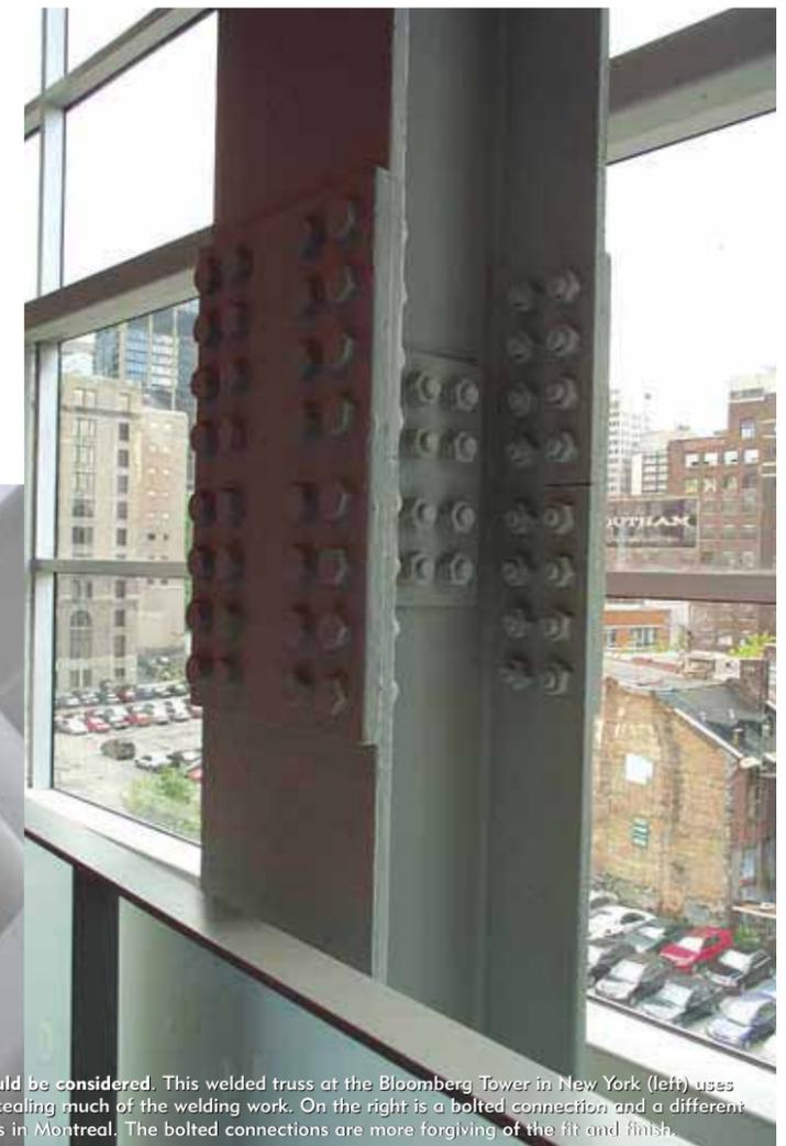
Tolerances of these fabricated forms are more stringent, generally to half of standard tolerance for structural steel. All of the surfaces would be "glove" smooth. The cost premium of these elements would be high and could range from 100% to 250% over the cost of Standard Structural Steel – completely as a function of the nature of the details, complexity of construction and selected finishes.
